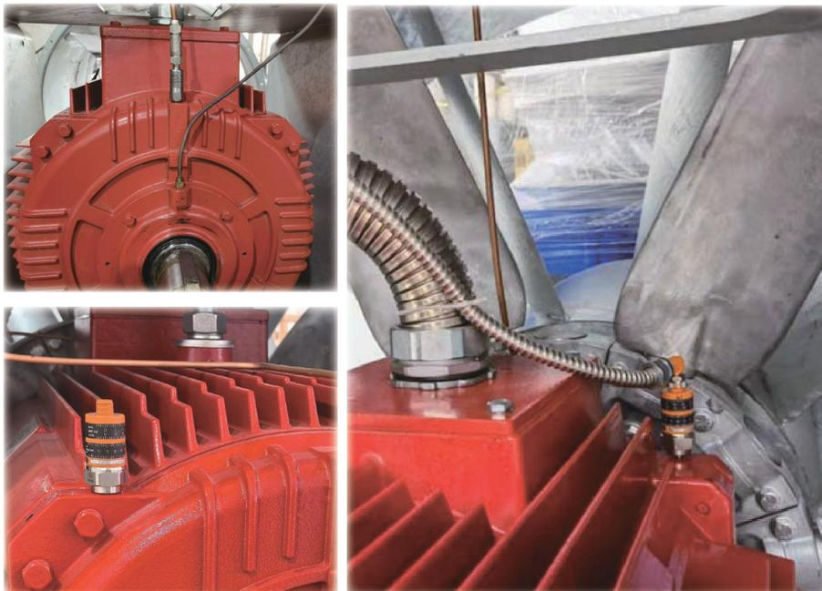
Note: Vibration Sensor should be installed at top of motor at drive end in vetical direction between -45 degree and +45 degree.
